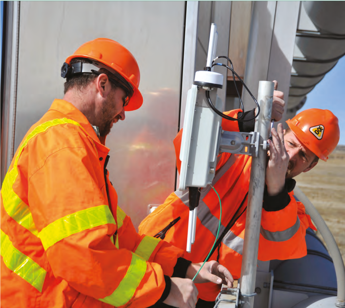
Left: DSRC roadside units are being installed in Wyoming to transmit workzone warnings to connected vehicles
