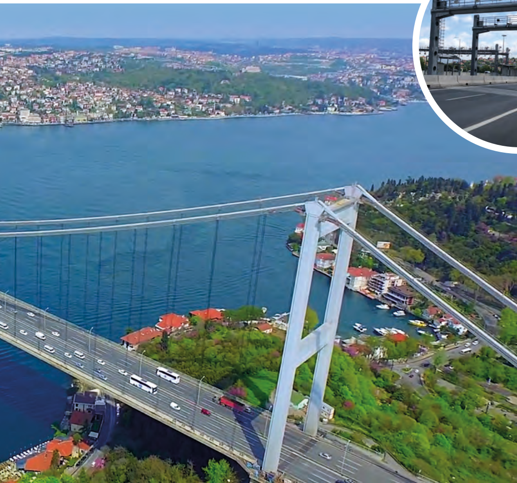
Far left: The Eurasia Tunnel is beneath the Bosphorus Strait
