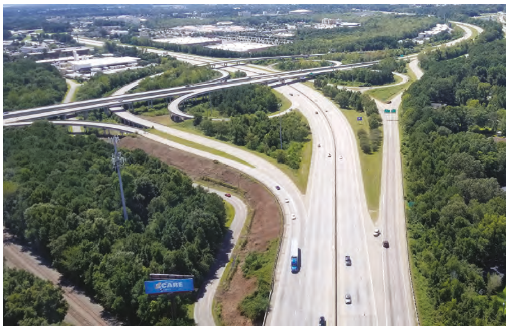
Left: Freeway capacity is doubled – but only in one direction – as a full-scale lane reversal trial takes place in South Carolina
