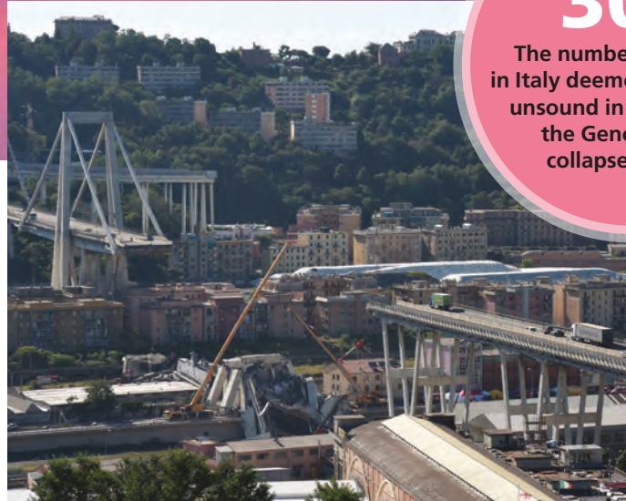
Left and far left: In August 2018, 43 people were killed when the Morandi Bridge in Genoa, Italy, collapsed
