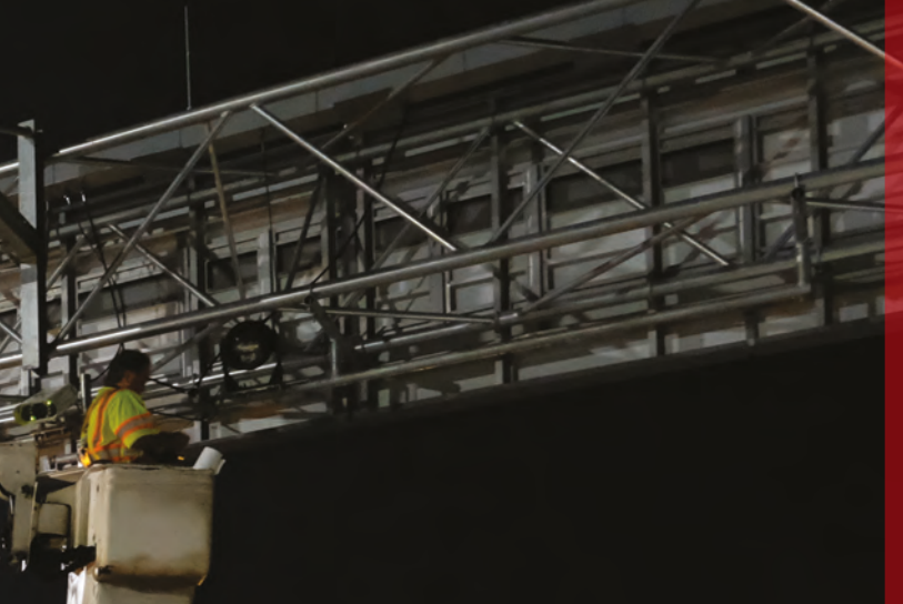
Left: The Triangle Expressway gantries were retrofitted with the new technology at off-peak times, to minimize disruption
