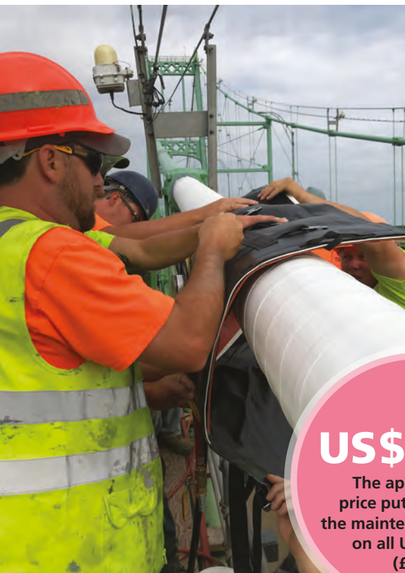
Left: The ‘Big Lift’ project involved the replacement of the road deck, floor beams, stiffening trusses and suspender ropes on the suspended spans of the Macdonald Bridge in Canada
