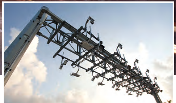
Above: SLAM allows the detection of subtle forms of system degradation
