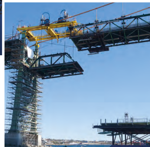
The refurbishment of Macdonald Bridge created some breathtaking sights
