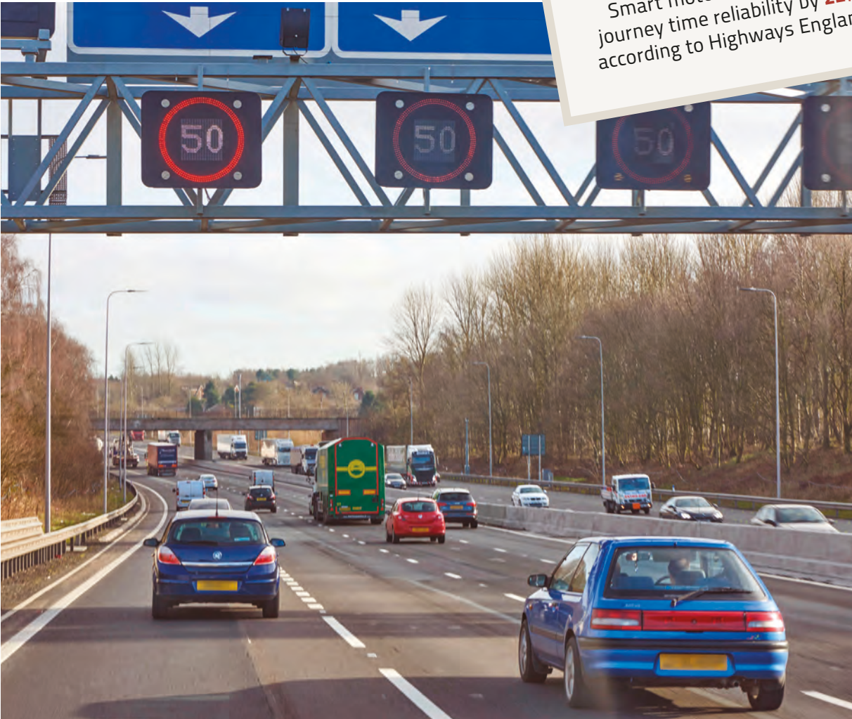
Left: Smart motorway algorithms use input from radar or buried magnetic induction loops to recommend variable speed limits
