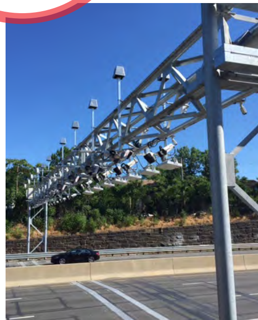
Above: One of the new multiprotocol-enabled gantries installed by Raytheon for MassDOT
