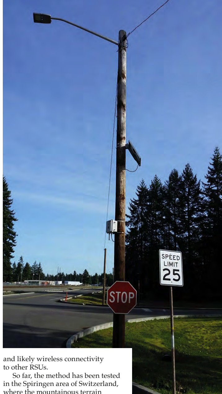
Above: A solar-powered Bluetooth detection unit attached to a telegraph pole in Washington
