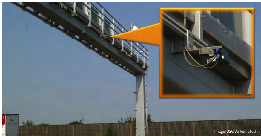
Overhead detectors can be neatly mounted right above the lane for maximum accuracy
