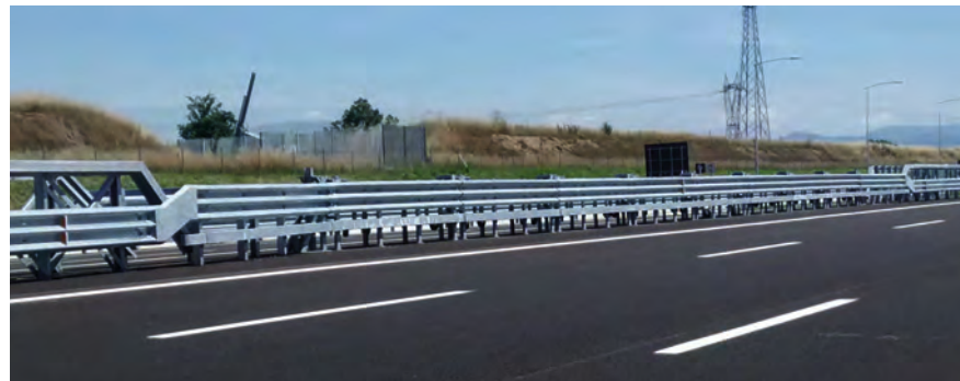
(Left) S-A-B system installed on the A54 in Italy
