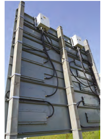
(Above left) The new M6toll signs show the current prices, and the next time period and prices (Above) The signs mount directly onto existing posts
