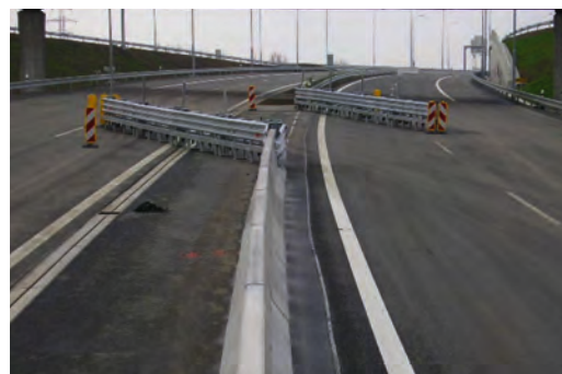
(Left) Installation of a S-A-B system in Slovakia
