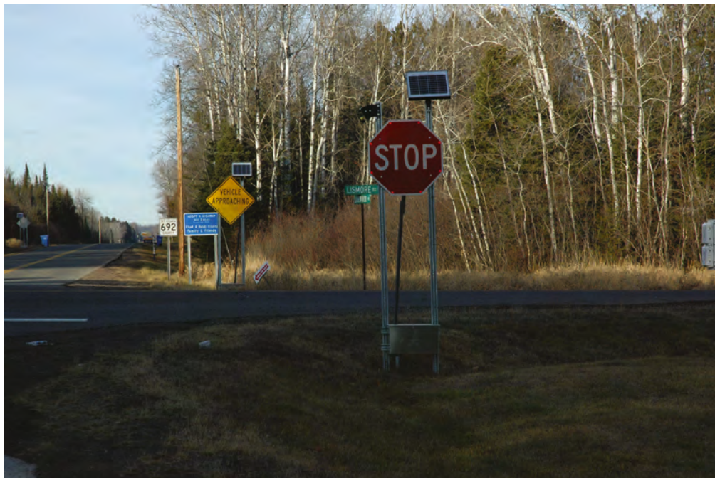
(Above) The ALERT-2 system installed in Minnesota
