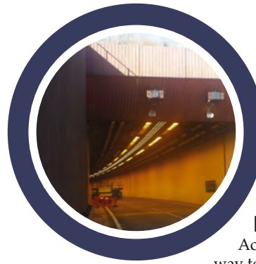
(Above) The Conwy tunnel prior to refurbishment
