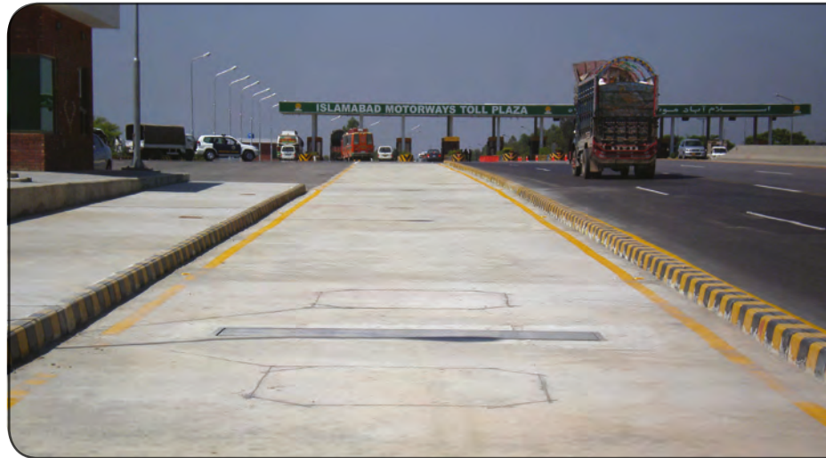
(Above and right) In Pakistan, high-speed WIM is not an option due to the associated costs, but some low-speed applications are in place
