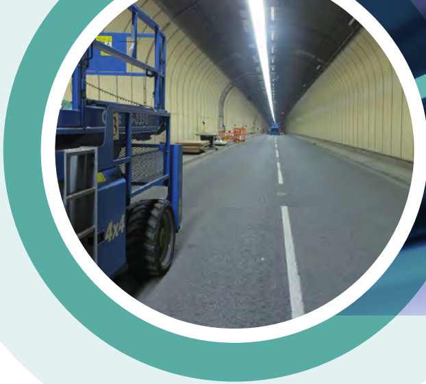
(Above) New LED luminaires in Pen-Y-Clip tunnel
