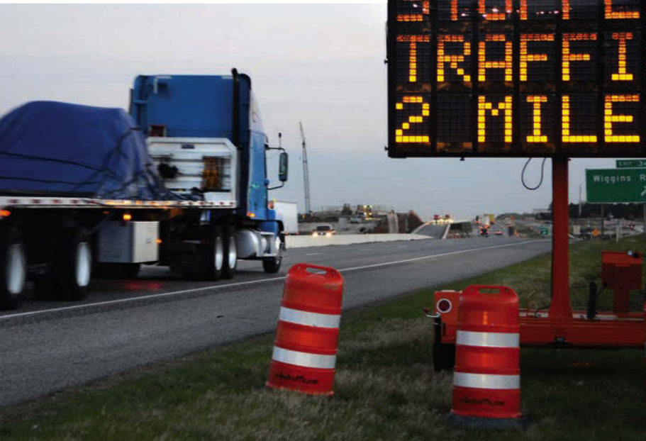
(Above and above right) Real-time queue warning VMS systems at workzones in Texas
