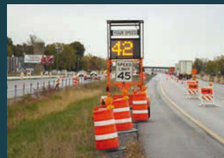
(Left) Nighttime workzones are dangerous places (Below) Illinois DOT has shown that queue and speed detection systems improve safety
