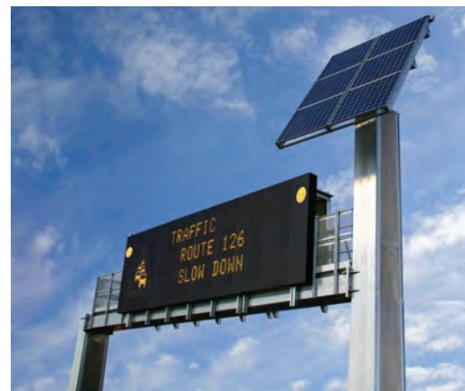
(Above left) A solar-powered safety DMS (Above) A traffic warning sign on a gantry (Left) A travel time DMS in Cape Cod
