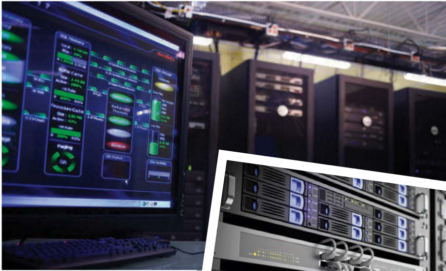
(Opposite) Mobile enforcement unit with integrated intelligence (Left and inset) Kapsch's Back Office software works with modern IT and communications infrastructure
