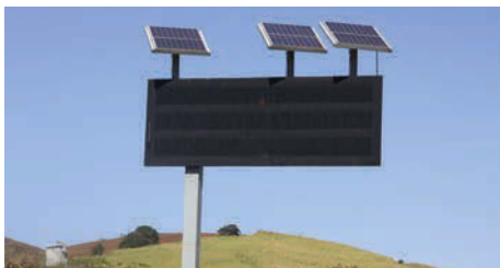
(Left) In South Africa high levels of solar radiation mean, in some areas, even large VMS can be operated without a traditional power source
