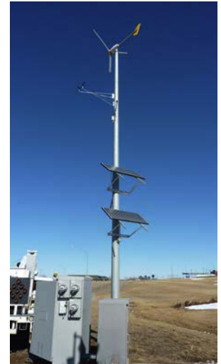
(Above) The solar/wind hybrid back-up power system being trialed in Lincoln, Nebraska
