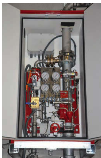
(Above) A water and foam system situated inside a fire-resistant cabinet
