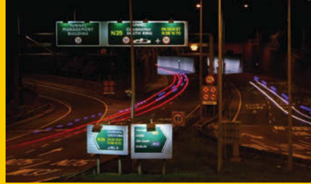
The Jack Lynch Tunnel is situated to the east of Cork city center
