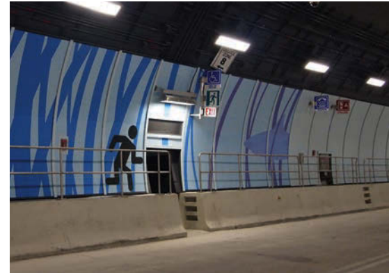
(Left) CCTV cameras monitor the traffic in the Port of Miami Tunnel 24 hours a day (Right) The tunnel's emergency exits are clearly marked and provide a refuge area for people with restricted mobility
