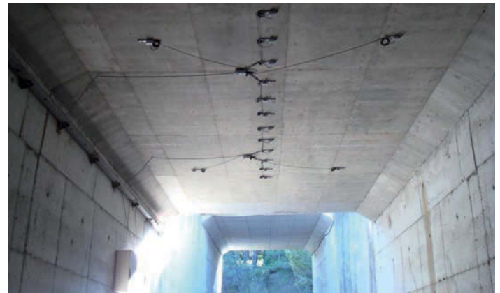
(Right) Bridge WIM systems are lightweight and easy to move between different locations
