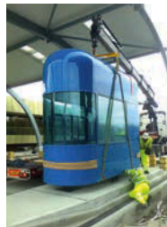
The new toll booths were installed under the new canopy in February 2014
