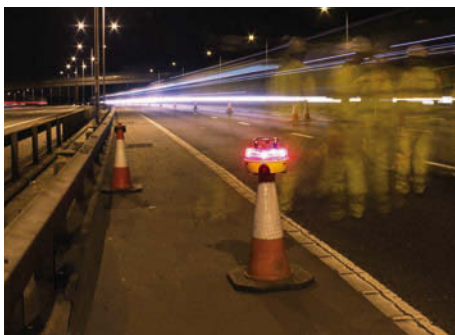
Intellicone enables standard traffic management equipment to be turned into an electronic safety perimeter
