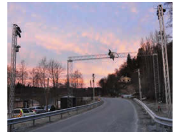
(Main) ETC relies on gantry-based equipment that must be available at all times (Below) Free-flow toll technology must have redundancy built in
