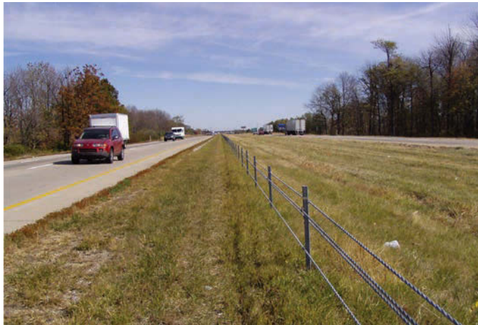
(Left) Cable barrier systems have been proven to help prevent accidents where vehicles cross the median and into other lanes of traffic. GIS helps determine suitable locations for their usage
