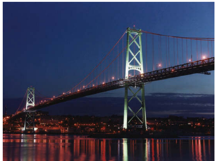
(Above) Beginning in 2015, the bridge road deck, floor beams, stiffening trusses and suspender ropes will be replaced on the Angus L Macdonald Bridge (Right) Figures from 2009 show that Halifax’s A Murray MacKay Bridge had an average of 52,000 vehicle crossings a day
