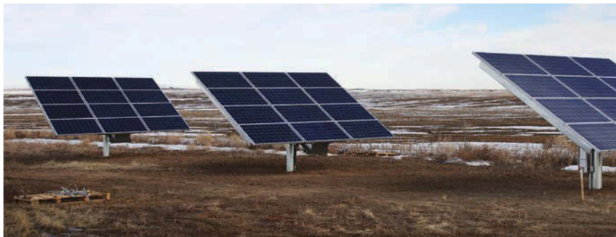
E-470 installed a network of solar-electric panels to power its signage (left) and its headquarter building (top)
