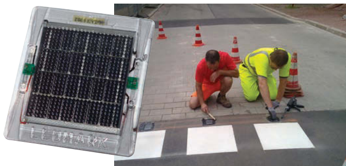
(Left) Dutch suburban and rural areas benefit from networks of safe and convenient cycle paths (Below) Geveko's LED-Mark lights being installed
