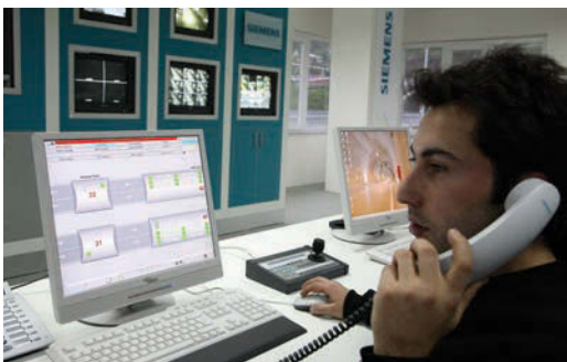
(Left) All the control and monitoring processes of the 29 tunnels are coordinated from the Trabzon TOC (Above) Systems from Siemens can recognize any traffic flow disruptions and activate alarms as necessary
