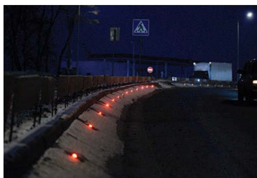
(Main) SR-20C studs in operation (Left) Studs can also be used to warn of ice
