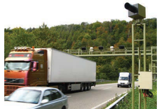
Section speed control is operating well in Switzerland but privacy issues have hindered its deployment in Germany
