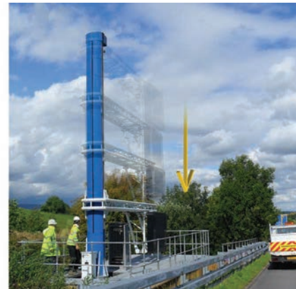
Crown International's VMC Pole is a rotating and lowering cantilevered pole – a smart solution for easier access to highway equipment
