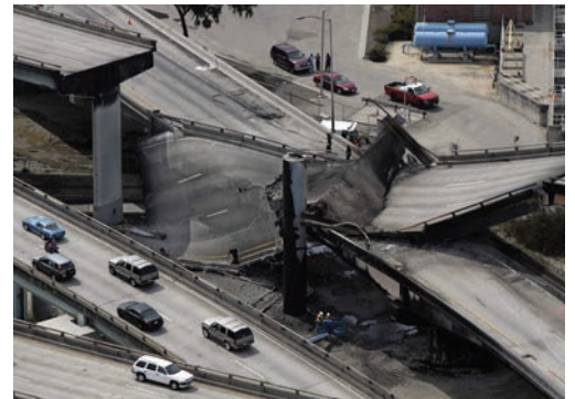
In April 2007, part of I-580 in Oakland, California, collapsed as a result of a fire started by a gasoline truck that crashed
