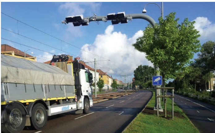
Q-Free's single gantry features two Prosilica GX1920 digital cameras by Allied Vision Technologies
