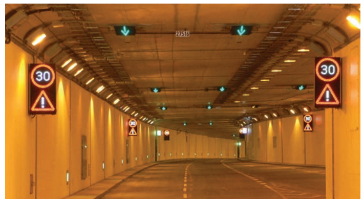
(Figure 1, below) Safety-critical application of VMS in a tunnel (Table 1, bottom) Fault classes and corresponding measures
