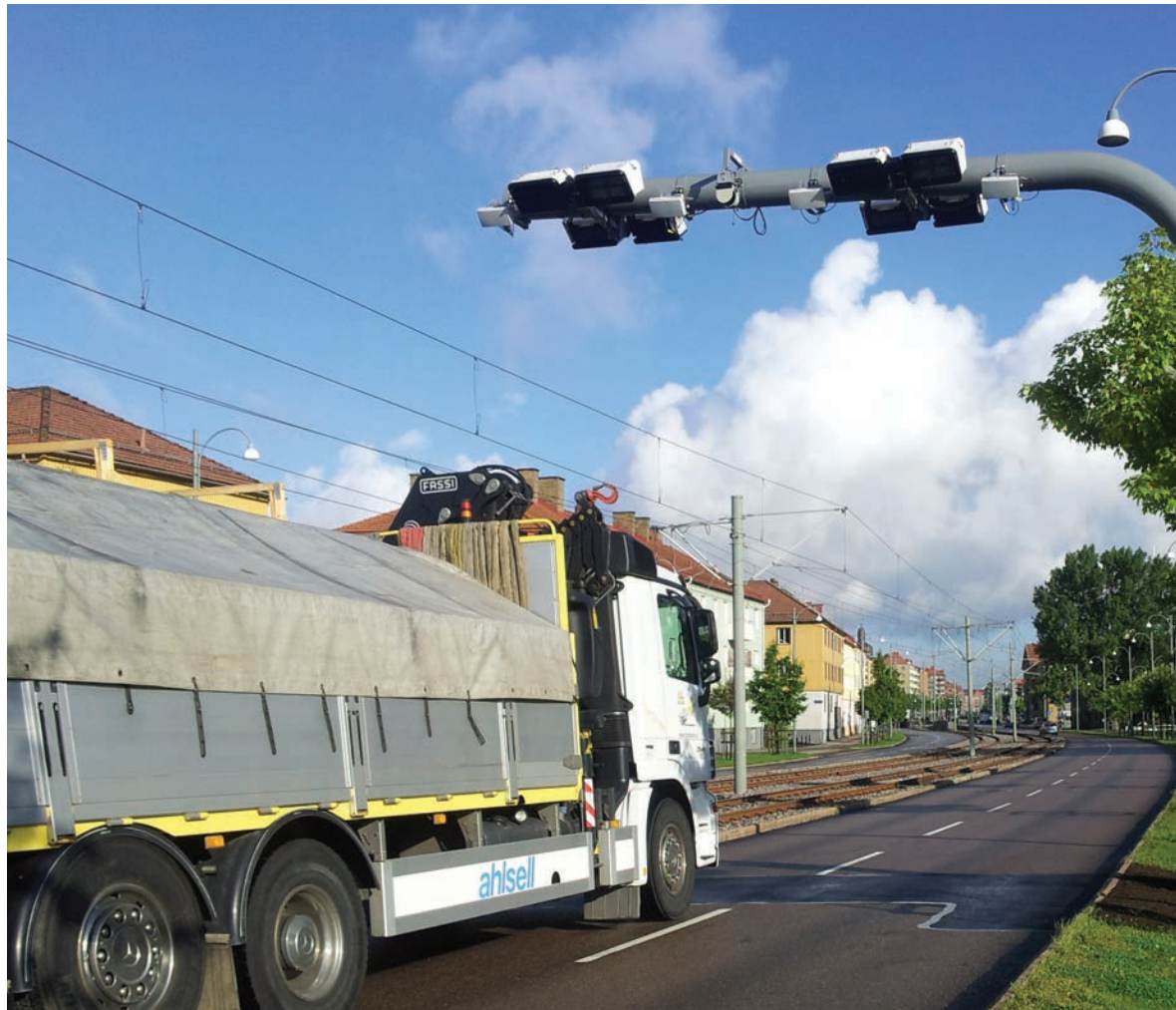
The single-gantry solution uses the latest imaging systems for ALPR
