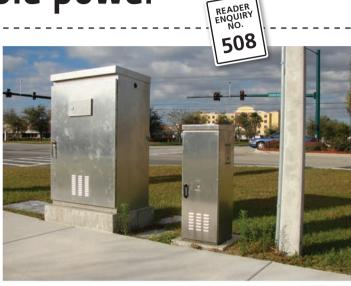
(Above) Alpha battery back-up system (small enclosure in center of photo) in operation in Port St. Lucie, Florida, USA (Right) Alpha outdoor traffic enclosure featuring UPS module and batteries
