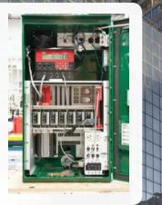
The TransSuite traffic management software is integrated with Encompass RFID readers, microwave sensors, the adaptive control module, and other related equipment using the NYCWiN. One of TransSuite's roles is to control the ASTC controllers wirelessly. RFID readers for data capture were supplied by the same vendor, which assisted NYCDOT with traffic controller specification development, procurement and testing, as well as with the NYCWiN wireless router procurement.
