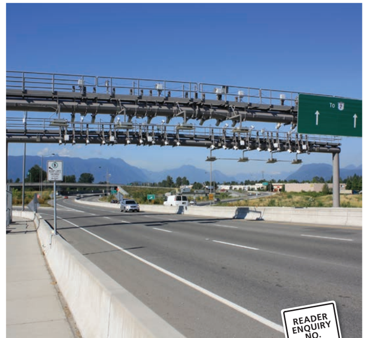
The Golden Ears Bridge, Vancouver BC, will be fully interoperable with the future Portmann Bridge free-flow system
