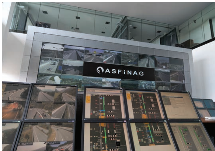
At ASFINAG's HQ data from both mobile and roadside sources will be collated
