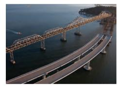
standard has now been created for bridges in California called 'Lifeline', which was really the first step in determining the design. Not only is there a no-fail or no-collapse criteria after a major earthquake, but the structure needs to be accessible, immediately, to the emergency services and for the post-event rebuilding effort. It's also stipulated they be returned to public service without being replaced."
