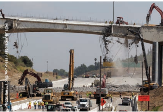
To accommodate an extra lane on the I-405, the Mulholland Drive overcrossing had to be replaced in phases
