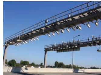
A variety of technologies, including ALPR cameras, is used to identify and classify vehicles
