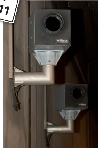
TraffiStar units deployed inside the Rennsteig Tunnel in Germany
