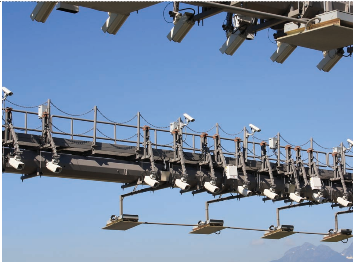
A variety of technologies, including ALPR cameras, is used to identify and classify vehicles
