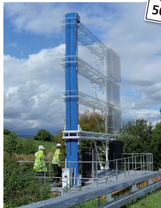
The VMC Pole helps with an array of traffic management tasks
