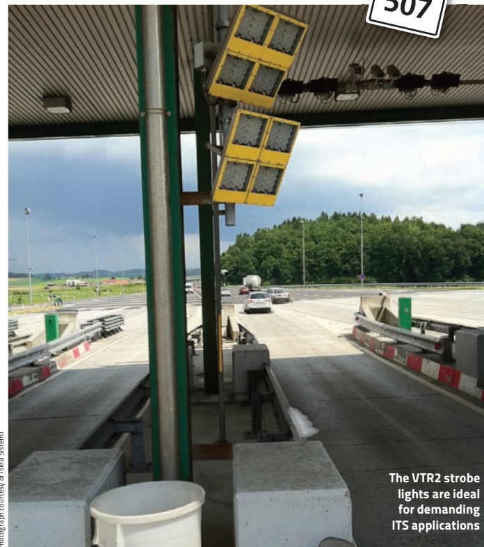
Photograph courtesy of Iskra Sistemi
