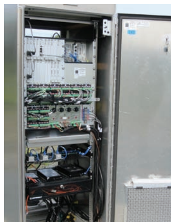
A weatherproof cabinet houses the iSINC
