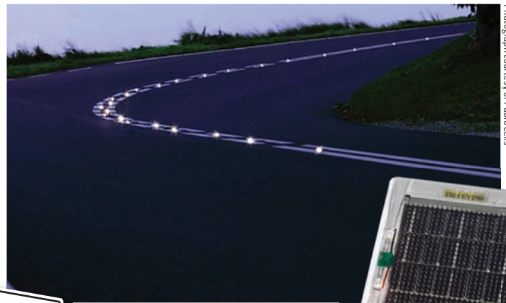
(Main image) Guiding lights in Aarhus (Right) Close-up of the LED-Mark (Bottom left) Geveko's LED-Guide
