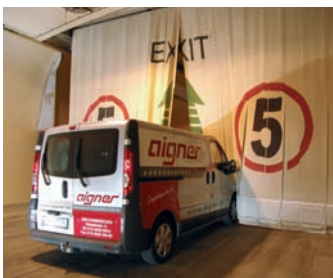
Fire curtains promote visibility and instruct drivers how to behave safely
