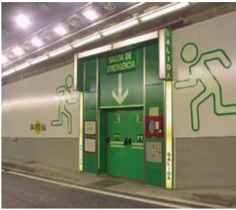
Tunnel exit signs are increasingly using IPT lighting for its safety merits
