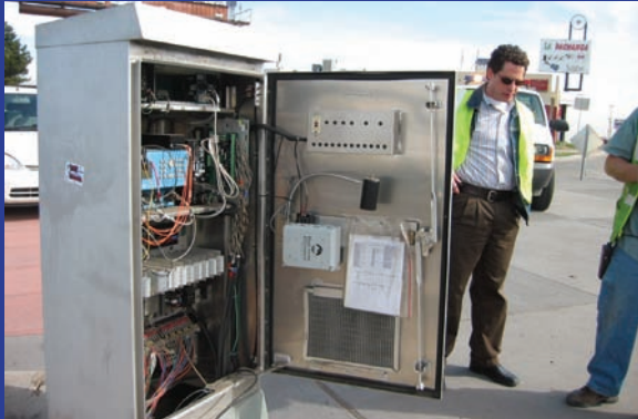
High Sierra Electronics installed pavement sensors at strategic locations on intersections in Denver
