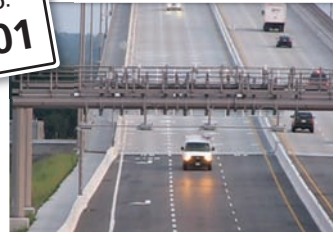
(Left and below) CS equipped the Golden Ears Bridge with a free-flow system that uses either a vehicle's Quickpass tag or video tolling in order to charge for payment
