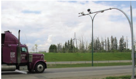
(Above) Close-up of IRD technologies for the enforcement of overloaded trucks (Above left) The use of a virtual weighstation system benefits a transportation agency, the trucking industry, and the general public in many ways
