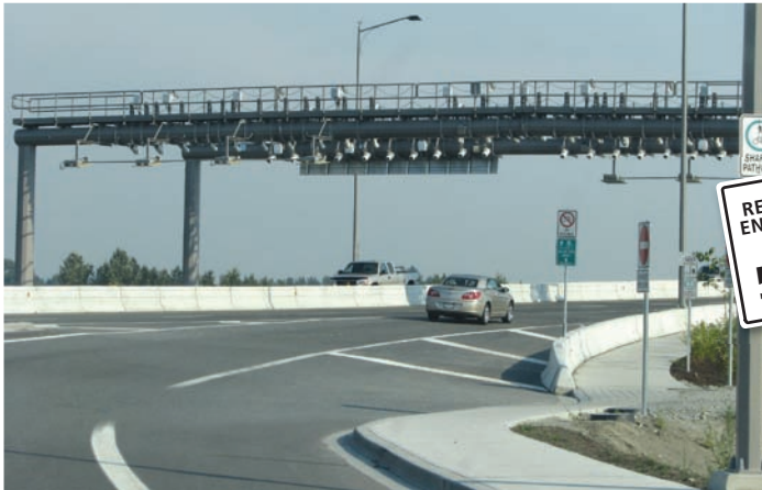
(Left and below) CS equipped the Golden Ears Bridge with a free-flow system that uses either a vehicle's Quickpass tag or video tolling in order to charge for payment
