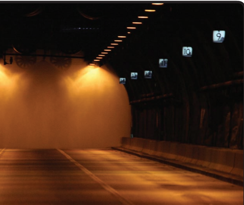
(Above) Deluge systems on the M5 East Sydney in Australia, which are a requirement in all Australian tunnel infrastructure (Left) Fire-fighting training in the Bonaventura Tunnel in Austria
