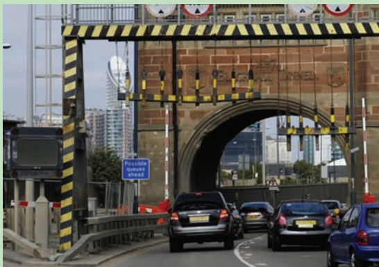
The VMS Limited solution is installed at the northbound section of the Blackwall Tunnel in London, UK
