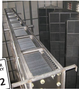
The Laerdal tunnel in Norway is taking advantage of CTA's electrostatic precipitator
