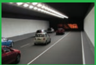
Linear LED tunnel lighting combines a flicker-free driving experience (exceptional uniformities) with outstanding visual guidance and excellent color rendering (white light)
