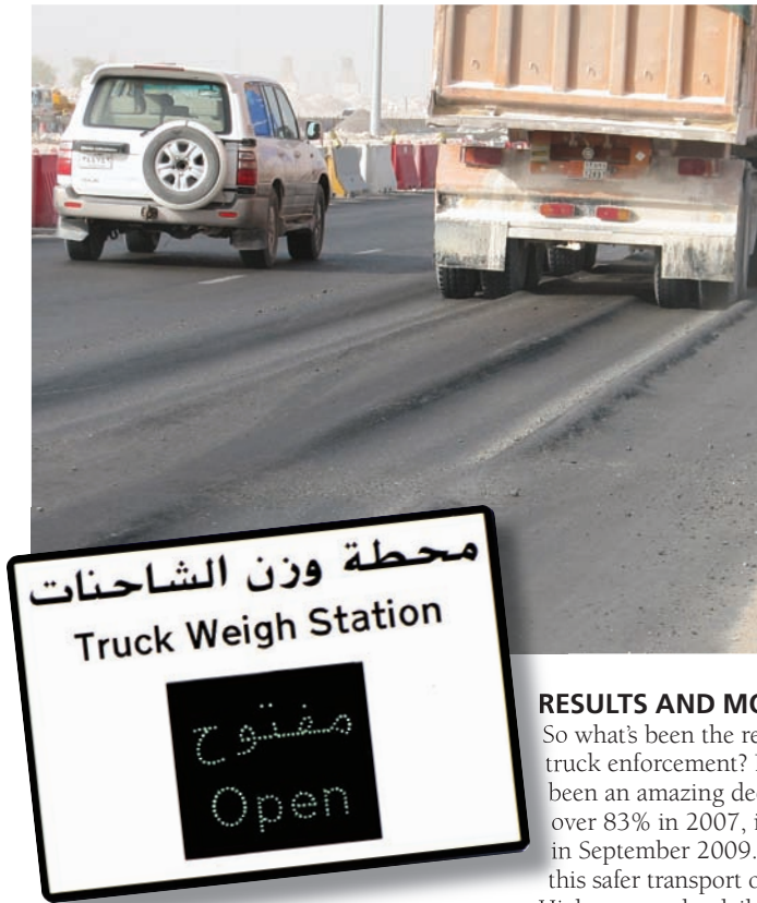
← Showing the damage – severe rutting – that overloaded trucks can cause to roads
