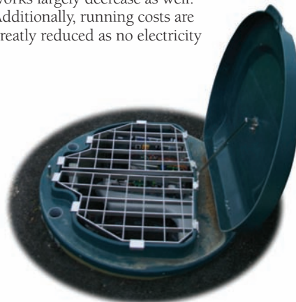
↑ The energy module, with batteries that store solar power, is buried in the ground
