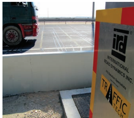
↑ Sensors embedded in the road capture information on vehicle gross weight, speed and axle classification
