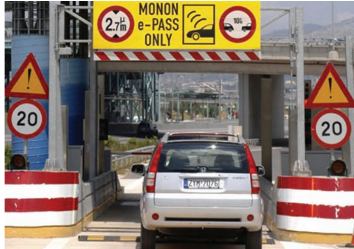
← Plazas on the Attica Tollway are equipped for both manual and electronic toll collection
