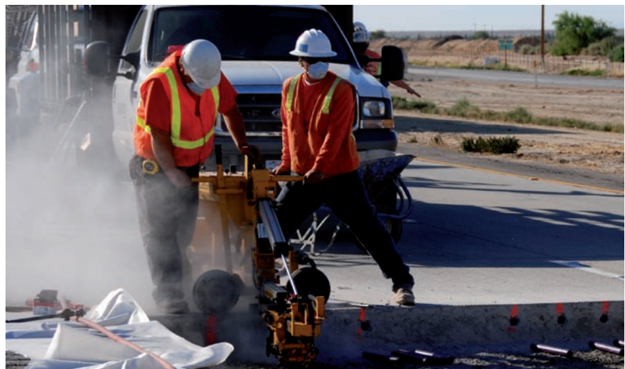
⊕ In times of limited funding, preservation and maintenance are key to conserving deteriorating roads
