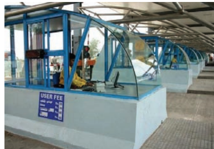
Ⓢ A tolling station in India, which features fiber-optic transmission equipment supplied by AMG
