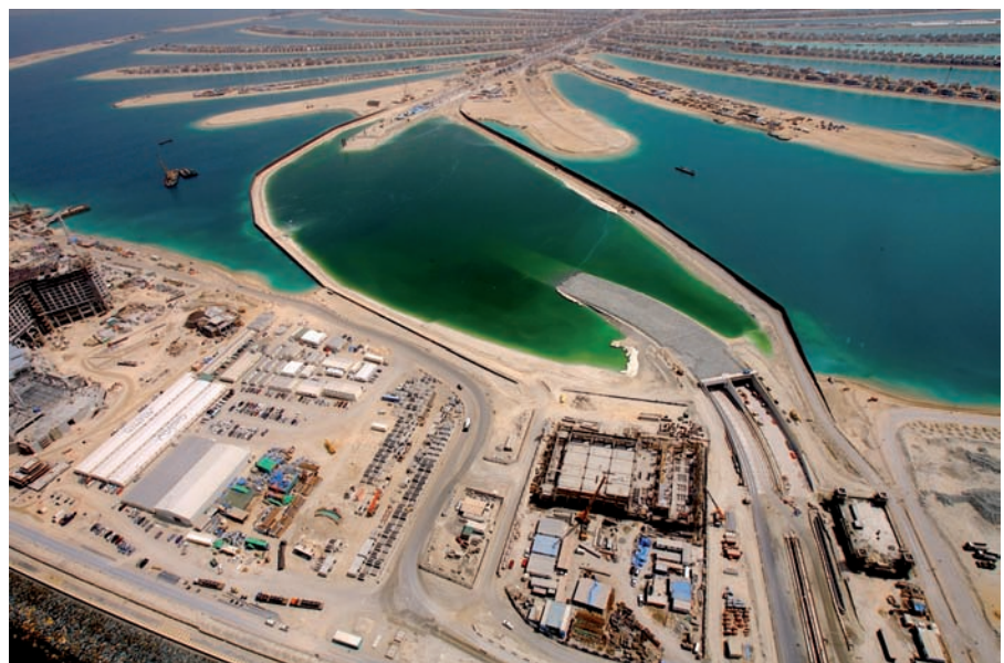
ⓘ The Palm Jumeirah tunnel in Dubai is a major engineering feat that required the installation of highly sophisticated video smoke-detection systems
