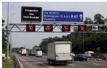
⬆️ One of the first hard shoulder running applications in the UK was part of an integrated ATM application on the M42 motorway
