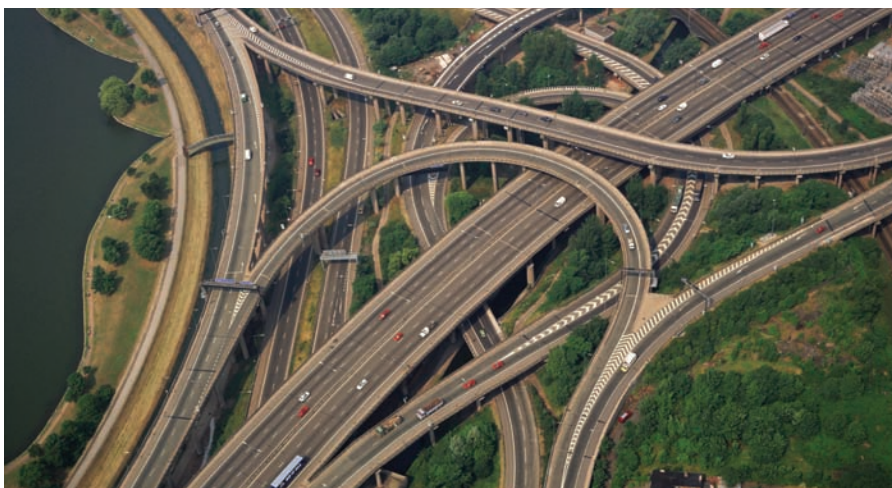
AMG was selected by the Highways Agency in the UK to develop a new network – the Birmingham Digital Ring – that would cope with traffic flows now and in the future in the busy Midlands area
