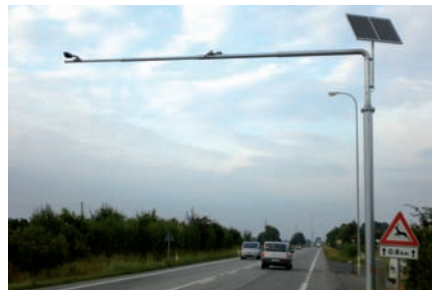
➤ Famas's Star C-500 can detect stationary and moving vehicles and classify traffic flows with an accuracy similar to an induction loop device
