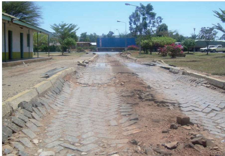
⤴ The costly and inconvenient pavement damage that is caused by illegally overloaded trucks
