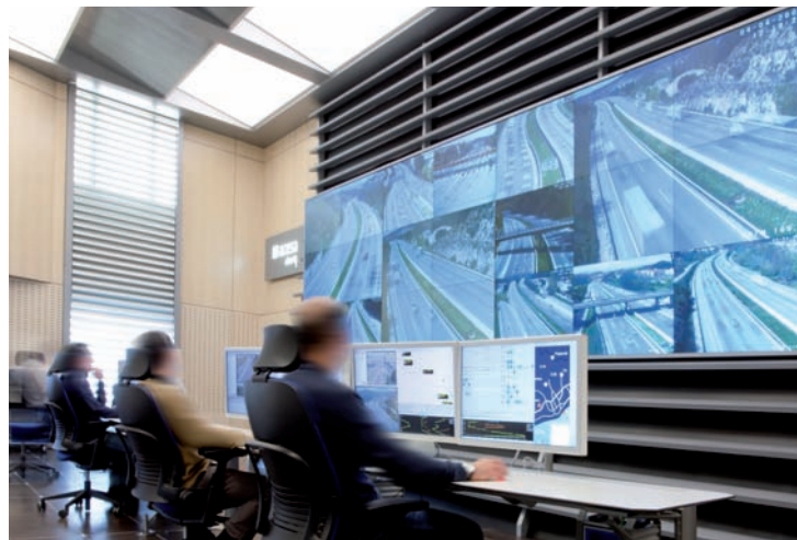
← The control room at Acesa Abertis's Barcelona TMC in Spain
