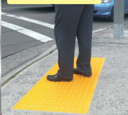
Pedestrian Switch Pads Surface mounted tactile pads for the directional and presence detection of pedestrians at crossings
