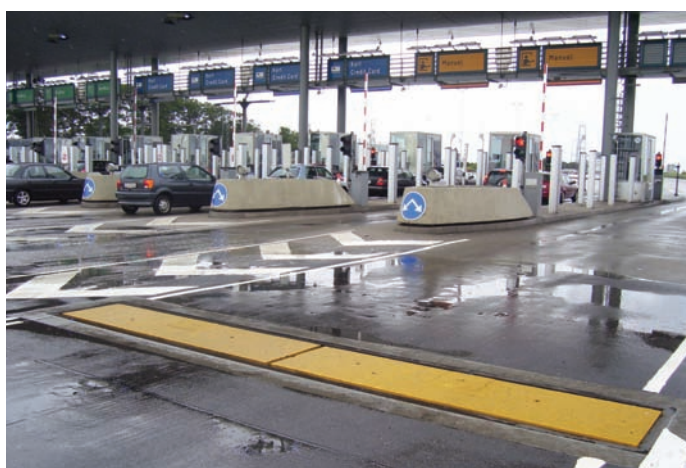
← The slower traffic at a toll plaza makes it the ideal location for weighing vehicles
