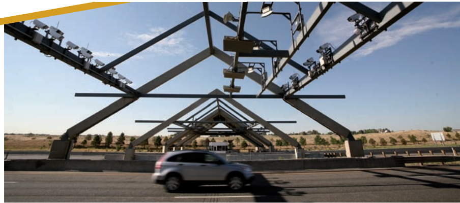
← Kapsch's mounted readers, vehicle detection and classification lasers, cameras and lights
