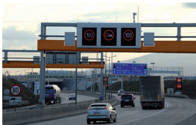
← Traffic control system on expressway S1, in Vienna, Austria
