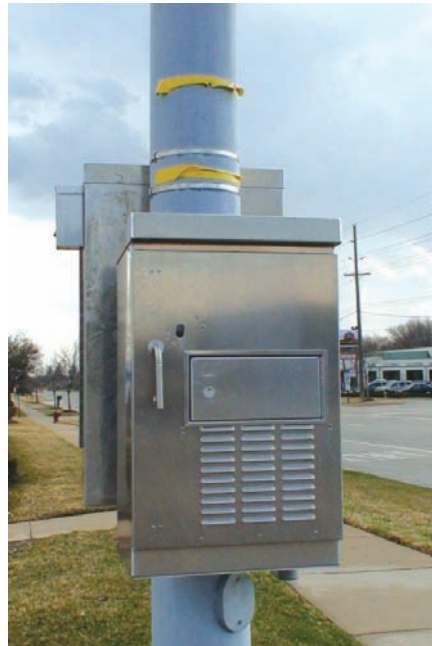
← RCOC signal controller/CICAS-V roadside cabinets
