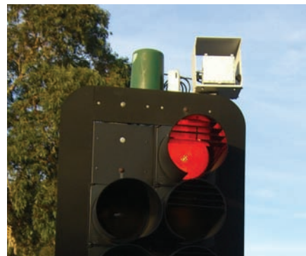
Example of Robot tracking radar installation using existing infrastructure
